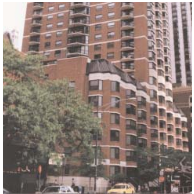
Residential units or other uses wrapping an enclosed parking structure allows the garage to be concealed from the street
