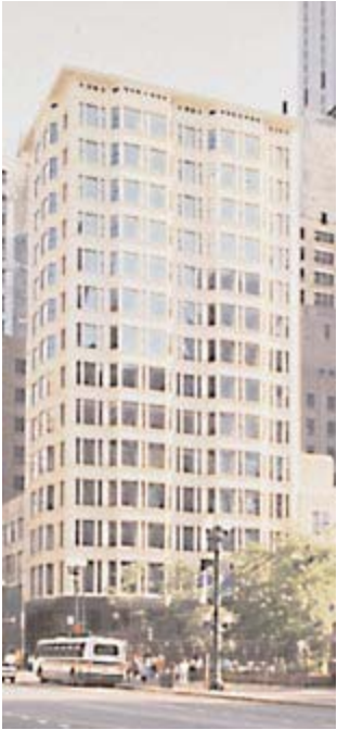
Reliance Building: conversion to Hotel Burnham underway
