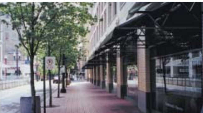
A parking structure with an attractive facade at the street level and above can maintain the attractiveness of the streetwall
