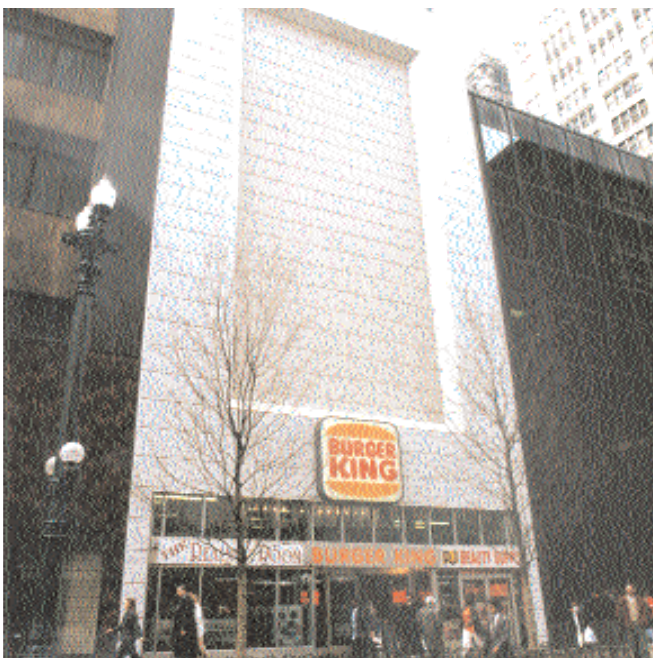
Inappropriate cladding should be removed to uncover and restore original building facades
