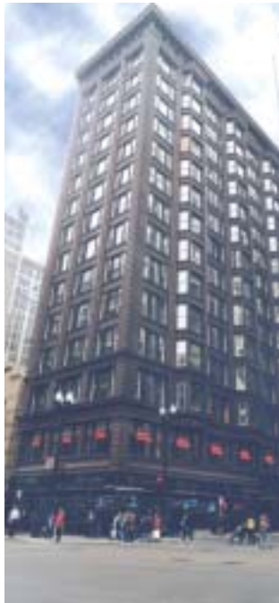
Chicago Building: dormitory for the School of the Art Institute of Chicago
